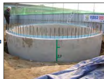
Install the caisson
