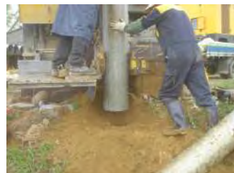
Casing installation
