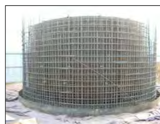
Install the rebar and reinforced concrete
