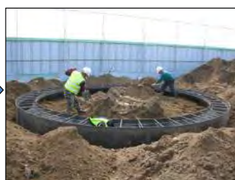
Install the sue steel sheet
