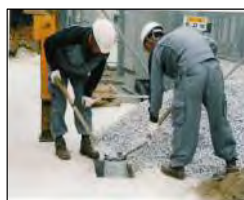
Insert backfill material into well
