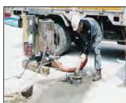
Impervious material injection
