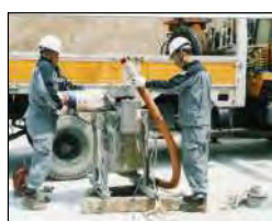
Impervious material injection
